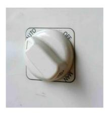
The diverter is installed with a 3-way changeover switch. This allows you to bypass the diverter in case the unit fails, needs to be turned off, or malfunctions.
